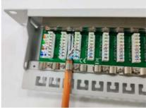
8. Apply the cable ties for strain relief and snap in the cover.
