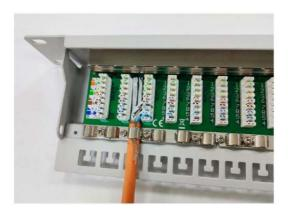
5. Cut the shielding foil to length.
